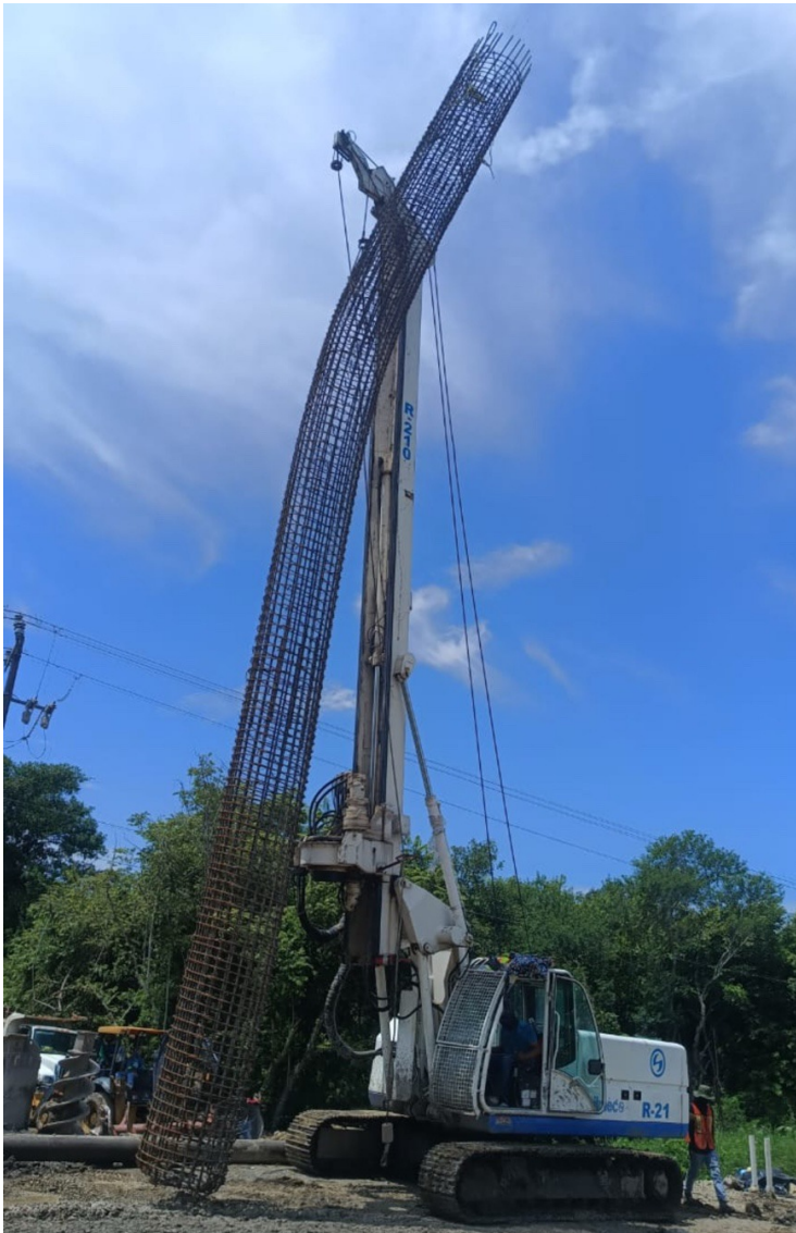
LIFTING OF LONG REBAR CAGES · SOILMEC R-210 · ROADSIDE WORK
