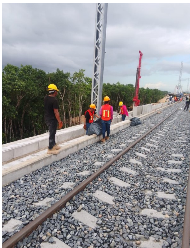
Erection of steel catenary posts.
