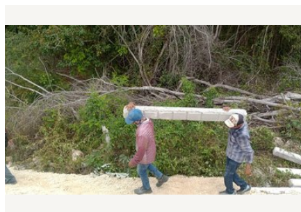
Transport to the work front.
